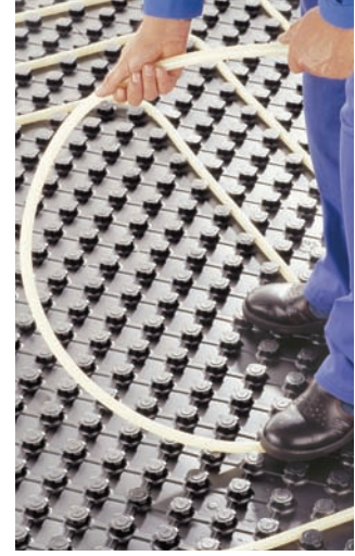
With the flexible pipes, shifts in direction during installation can be implemented in seconds.
